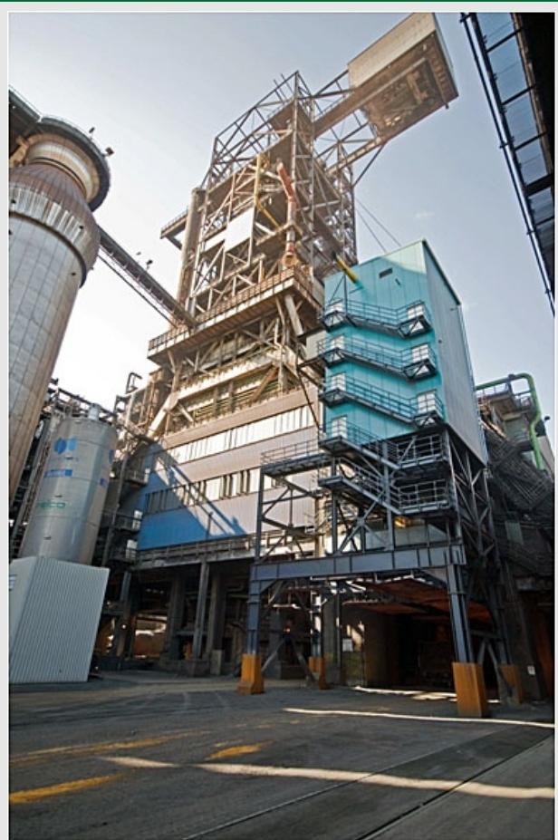
PCI+® V installation in front of the blast furnace
